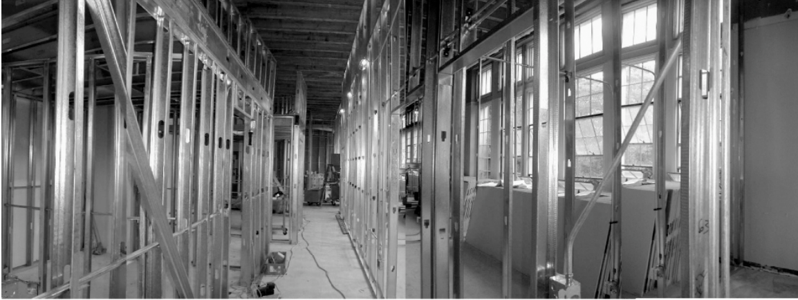
Raitt Hall Main Campus Construction and Build-out
