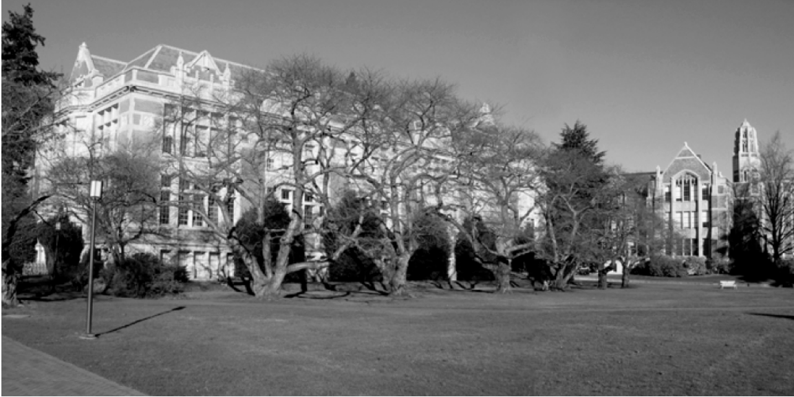
Raitt Hall Main Campus Laboratory, Classrooms and Facilities
