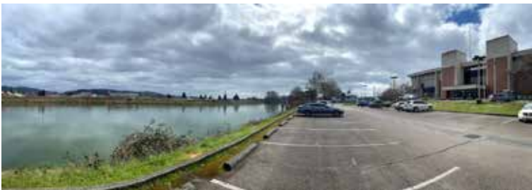
Figure 42: The Cowlitz River and the Cowlitz County Hall of Justice in Longview, WA
